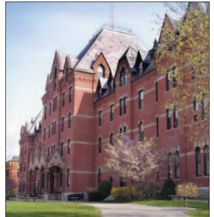
Dean College is saving more than $40,000 a year on energy bills thanks to a Wilkinson-engineered solution that includes Autoflame technology. (Photo courtesy of Dean College)
