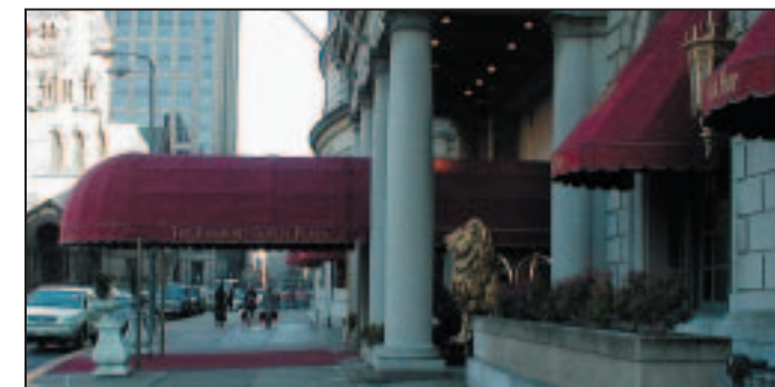
The Fairmont Copley Plaza Hotel, one of the oldest and most luxurious in Boston, upgraded its boiler plant by installing two Wilkinson Centurian™ steel firebox boilers featuring Autoflame advanced combustion technology.
